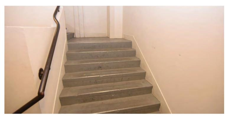
Photo of Stair 4 at level 10. A handrail would need to be added to the stair if the building is substantially altered. CDG photo, May 7, 2016.
