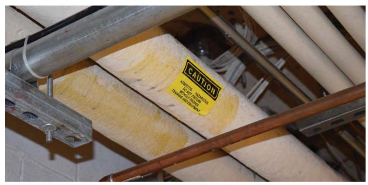
View of label identifying asbestos pipe insulation. CDG photo, May 24, 2016.
