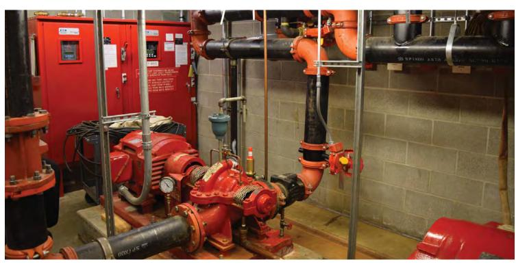
Photo of fire sprinkler pumps, fire sprinkler control panel, and fire protection water piping at basement Room WB9B. CDG photo, May 24, 2016.
