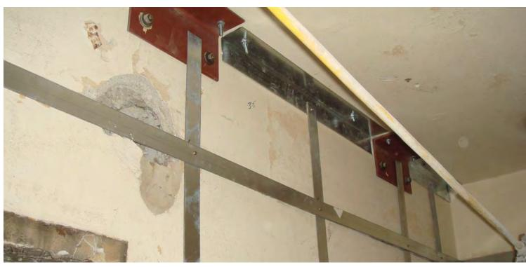
Example of steel strap strongbacking for hollow-clay tile masonry interior wall. CDG photo, April 22, 2015.
