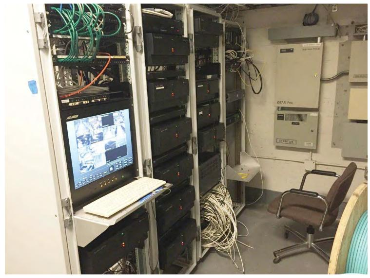
**FIGURE 4** Room CB40 - Feeds from security cameras are routed through Security Room CB40 in the basement before being fed up to Security Office E195
