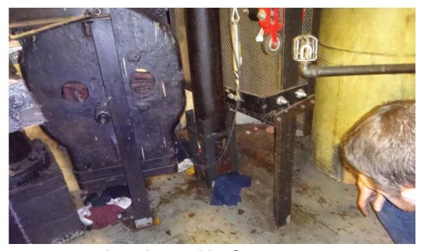
Figure 14 – Typical pit with rags and dirty floor.
