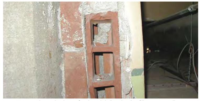
King County Courthouse, detail view of voids inside hollow clay tile infill at exterior walls. CPL photo, February 1, 2001.
