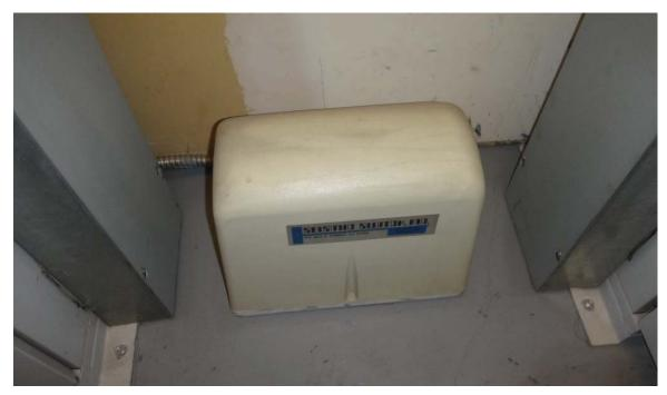
Figure 3 – Seismic switch installed during the modernization in 2004/05.
