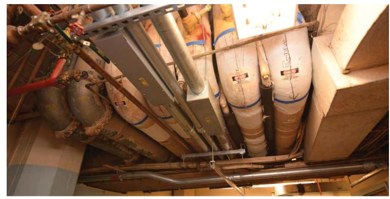
View of labels identifying asbestos pipe insulation. CDG photo, March 18, 2016.
