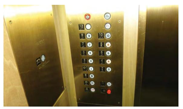
Figure 6 – Bronze fixtures installed in 2004/5 during modernization Meet code except for push/pull stop switch.
