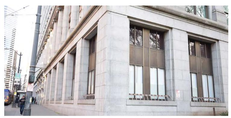
King County Courthouse exterior, view of the aluminum window wall systems at the southwest corner of the first floor. CDG photo, March 18, 2016.
