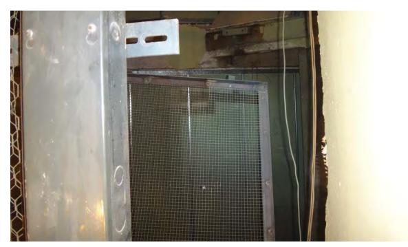
Figure 11 – Part of hoistway screening between Cars 9 and 10 is coming down and should be re-anchored.
