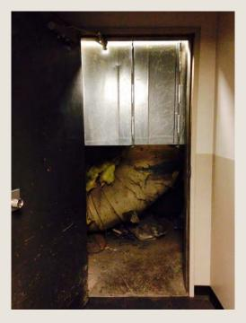
Figure 2 Access to floor 1A east electrical room by crawling under ductwork, a serious safety hazard and code violation
