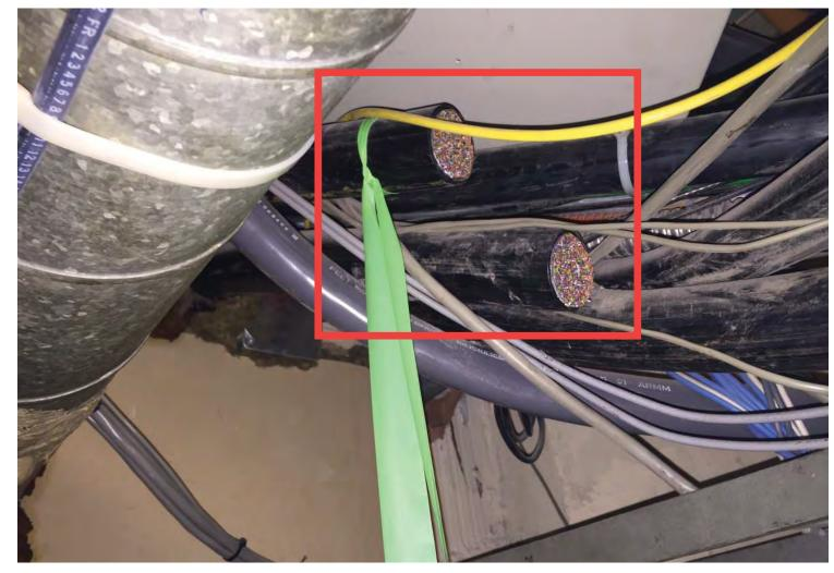
FIGURE 8 Communication cables have been severed and abandoned in place
