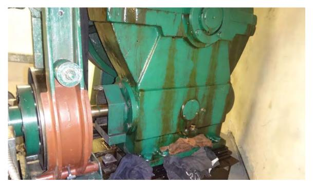
Figure 5 – Geared elevator machine for Cars 11 and 14 is leaking oil.
