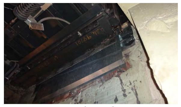
Figure 12 – Car aprons are missing from most of Cars 1 to 10.
