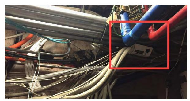
FIGURE 10 Communication cables are supported by electrical conduit
