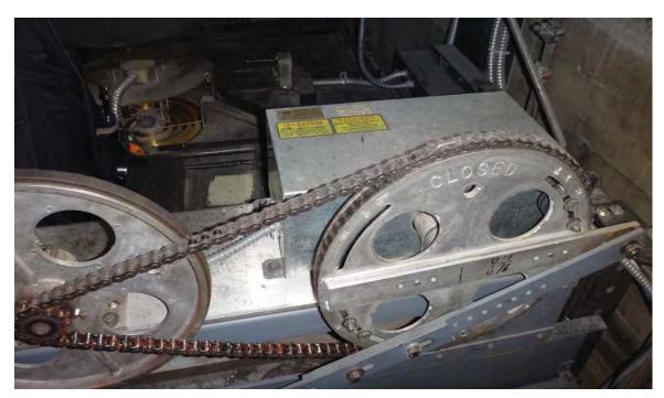
Figure 8 – GAL MOVFR closed loop door operators installed during modernization in 2004/5.
