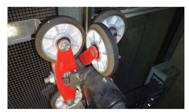
Figure 9 – High quality ELSCO roller guides installed during the 2004/5 modernization.
