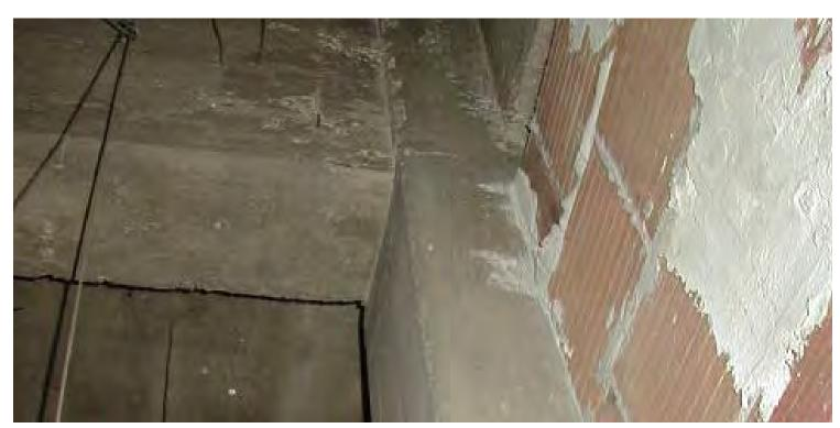
King County Courthouse, view of hollow clay tile infill between reinforced concrete columns at exterior walls. CPL photo, February, 1, 2001.
