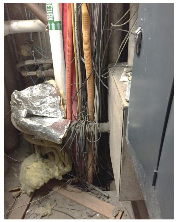
**FIGURE 9** Vertical cable run in mechanical chase. Abandoned and severed cables are run alongside operational functioning cables, along with construction debris. The National Electrical Code (NEC) requires removal of abandoned communications cabling
