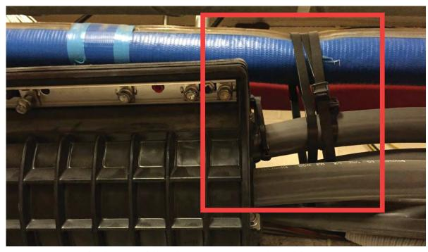
FIGURE 11 A telephone cable splice is supported by cold water piping
