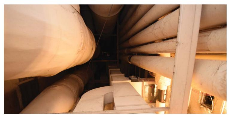
View of ducts and piping inside vertical mechanical, electrical, and plumbing shaft. CDG photo, March 31, 2016.
