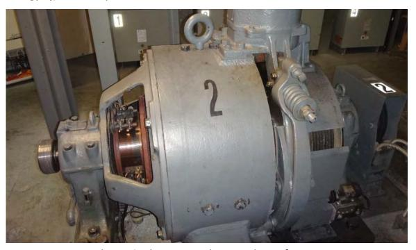
Figure 2 – Original Westinghouse Gearless machines for Cars 1-10 appear to have been installed during the 1960 modernization of the Court.
