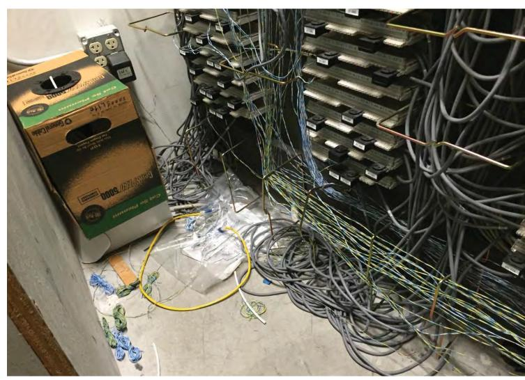
FIGURE 12 Proprietary low-density cable patching system. Debris from construction and maintenance has been allowed to accumulate in communication spaces
