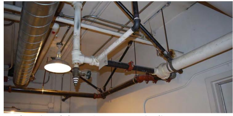
View of seismic bracing for fire protection water piping at ceiling of basement Room EB9. CDG photo, May 24, 2016.
