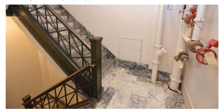
Photo of Stair 4 at level 5. The existing handrail is non-code compliant and may need to be upgraded if the building is substantially altered. CDG photo, May 7, 2016.
