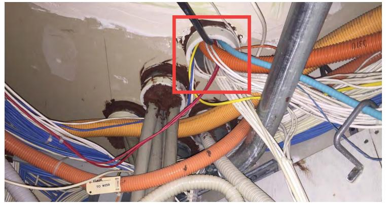
**FIGURE 5** Level 1 Intermediate Distribution Frame (IDF) - An example of typical floor penetrations. The two sleeves on the left have intumescent putty installed for firestopping. The sleeve on the right is missing firestopping on this level
