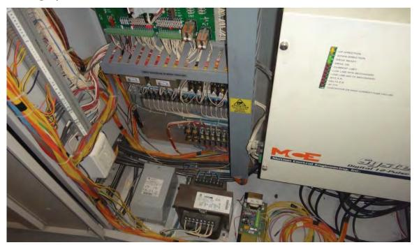
Figure 1 - Motion Control Engineering (MCE) IMC controllers with energy efficient 12 pulse SCR drives installed on Cars 1-10.
