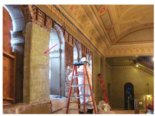
Example of fiberglass mesh strongbacking reinforcement for masonry walls. Photo from National Park Service Preservation Brief #41. Courtesy Wiss, Janney, Elstner and Associates.
