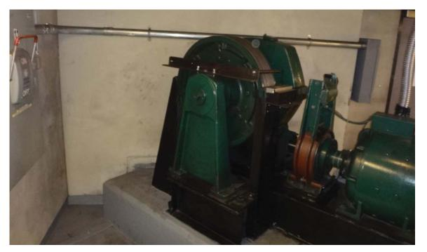
Figure 13 – Geared hoist machine for Car 11. Manufactured by Dover.
