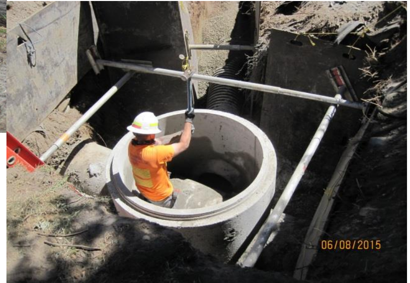
Below: Installing a new manhole at Seola Pond outlet.
