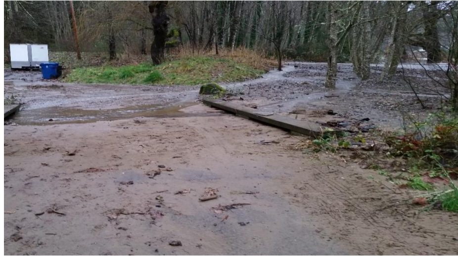
Burns Creek Channel Deposition and Flooding around Private Bridge
