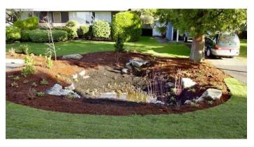
Create an inflow with a pipe or rock-lined ditch from your downspout to the upper edge of the rain garden. Protect that area with rock too.
