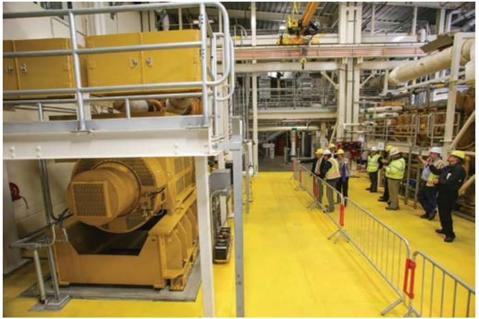
*The cogeneration facility at the West Point Wastewater Treatment Plant turns digester gas generated during the treatment process into electricity, which is sold as green energy in partnership with Seattle City Light, and heat energy, which is used onsite.*
