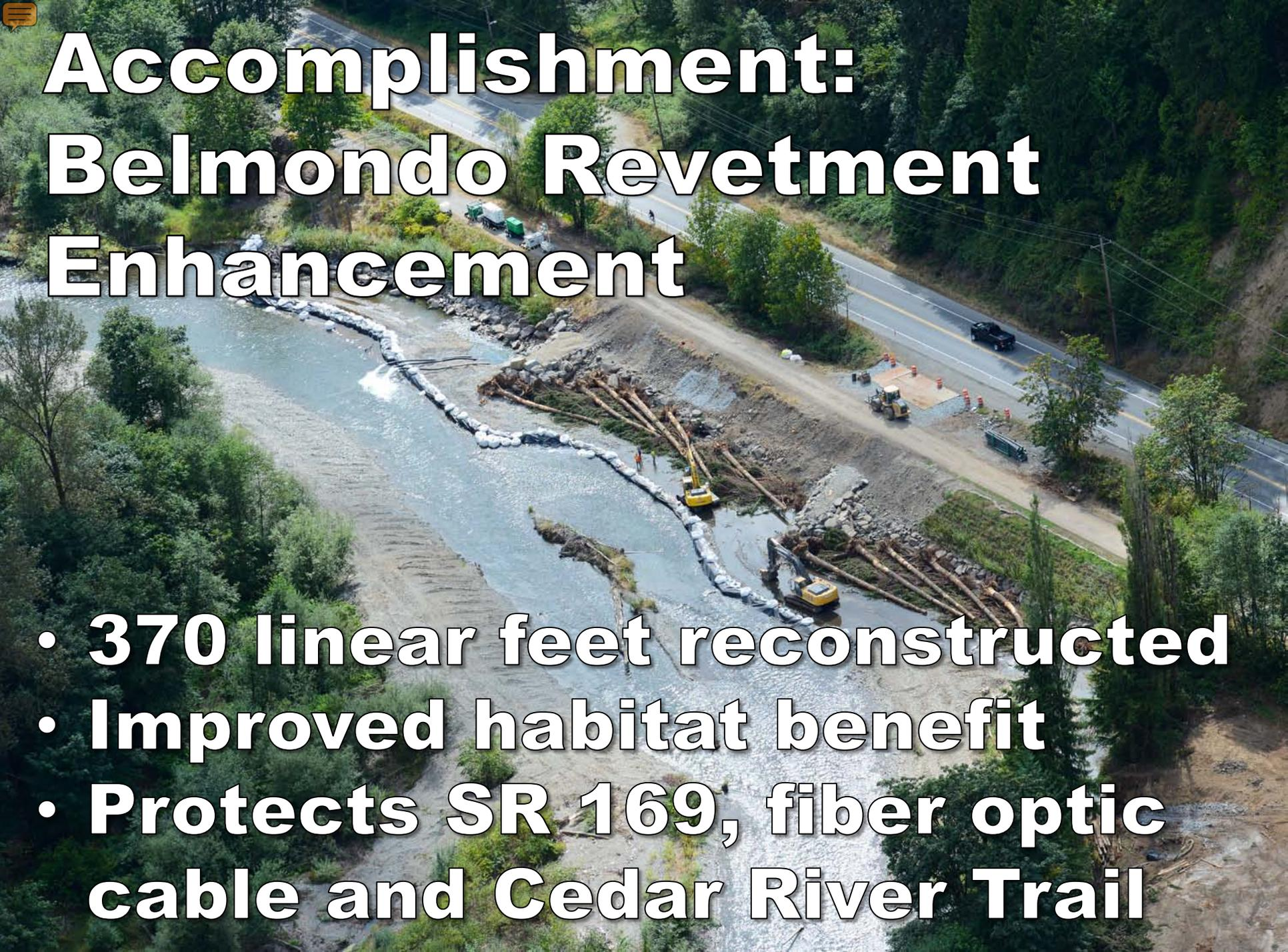
An aerial photograph showing a river construction project. A long line of white sandbags or silt curtains runs along the riverbank. Several yellow excavators are working in the water and on the bank. Large logs are piled up on the right side of the river. A paved road with a black car and a dirt road with construction equipment are visible in the upper right. The surrounding area is lush with green trees.
